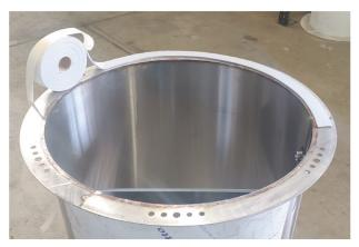
3. Install transition ring on top of intake using four (4) 1&½" stainless steel bolts, eight (8) stainless steel fender washers and four (4) stainless steel nuts. Apply foam tape to exposed side of poly transition ring.
