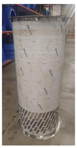
2. Once the intake section is completely positioned properly, install foam tape on top ring of intake section
